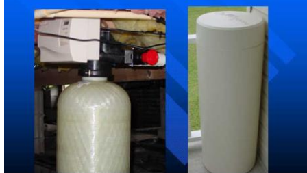
ION Exchange (Water Softener)
